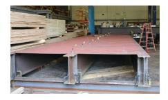
is fabricated mostly offsite and can be erected 30% to 50% faster than a traditional concrete-on-metal-deck floor system. It was launched as part of AISC's 2019 Need for Speed initiative, which aimed to design and construct steel buildings 50% faster by 2025 (a goal the industry achieved ahead of schedule).
